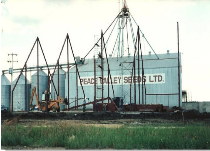
Constructing storage shed at original Peace Valley Seeds plant.
